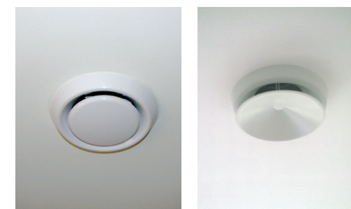
Ceiling-mounted extract and supply terminals (MVHR)
