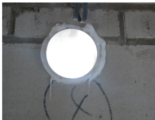
Stub duct for a through-the-wall fan with air tight seal to surrounding masonry
